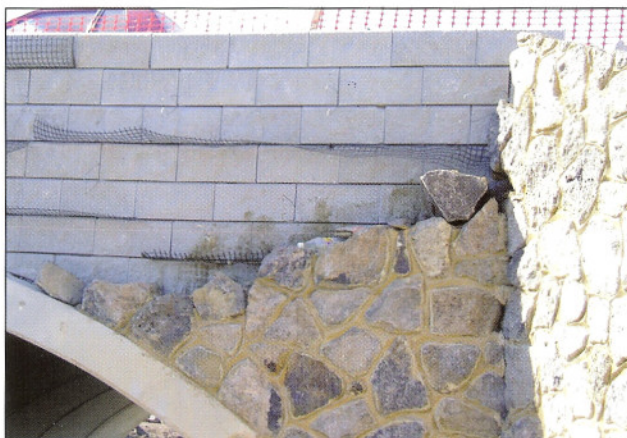
Mortared split rock-stone pitching with ties
