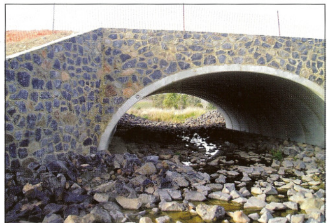
Completed culvert head and wing walls
