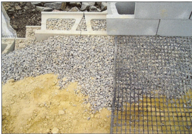
Allan Block and Miragrid 5XT geogrid
