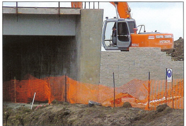
Bridge approach retaining wall under construction
