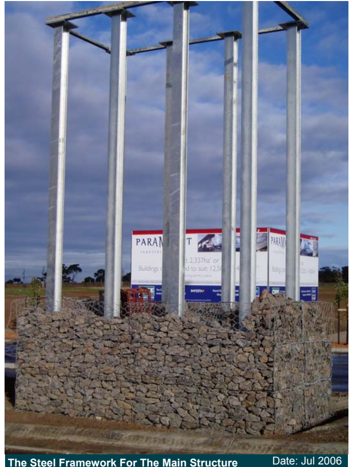
The Steel Framework For The Main Structure Date: Jul 2006
