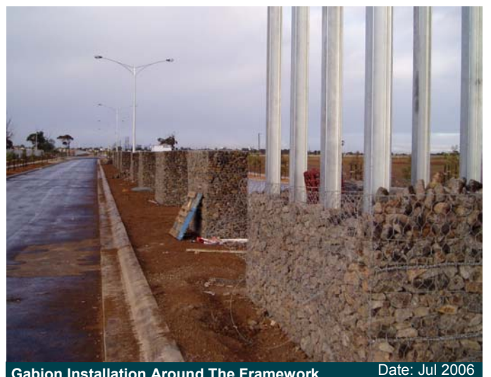
Gabion Installation Around The Framework Date: Jul 2006
