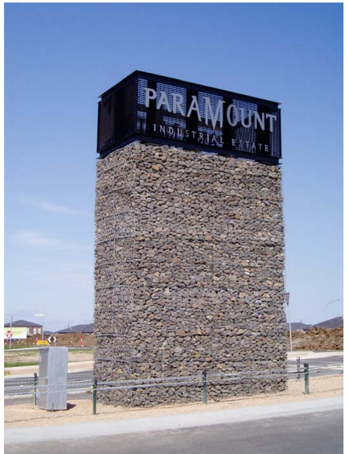
Large Feature Completed
