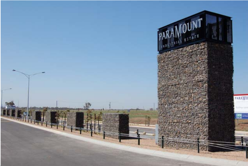
Large Feature After Construction
