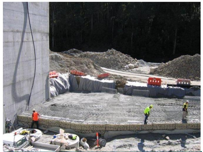
Gabion Facing With Woven Mesh Soil Reinforcement
