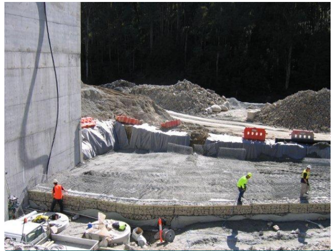
Gabion Facing With Woven Mesh Soil Reinforcement
