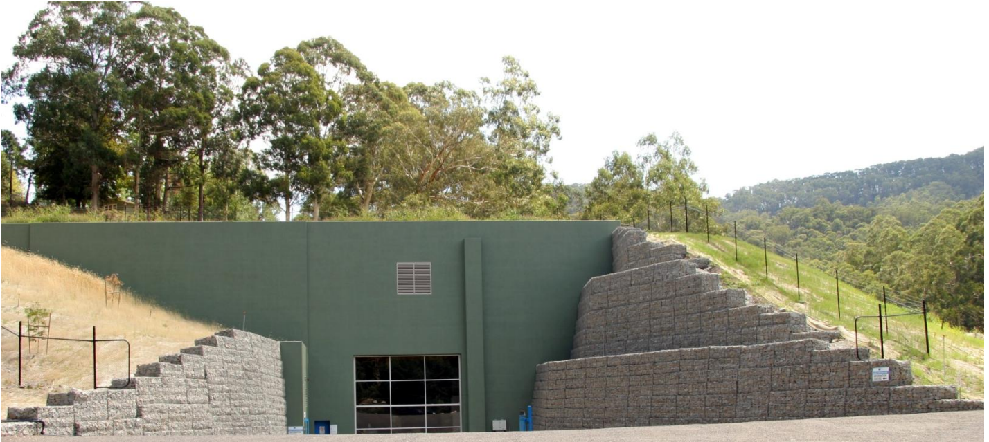
The Terramesh Walls At The PowerStation Entrance
