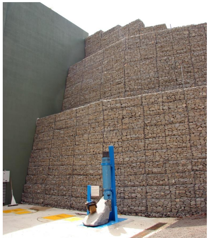
The Completed 15m High East Wall
