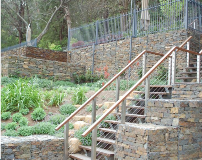
Terraced Walls With Vegetation
